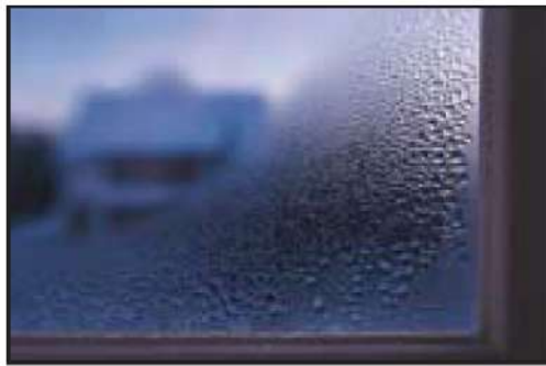
Condensation on the inside of a windowpane.
