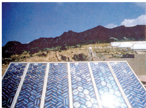
(a) This is a solar cell panel. It has a large number of solar cells joined in series
