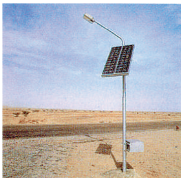
(b) A street light working on solar cell panel
