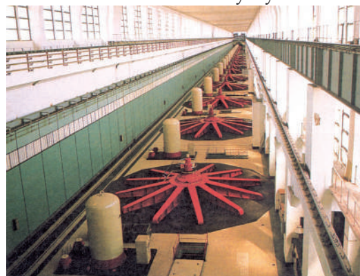
Figure 18. The turbines inside a hydroelectric power station which rotate by the force of fast flowing water.
