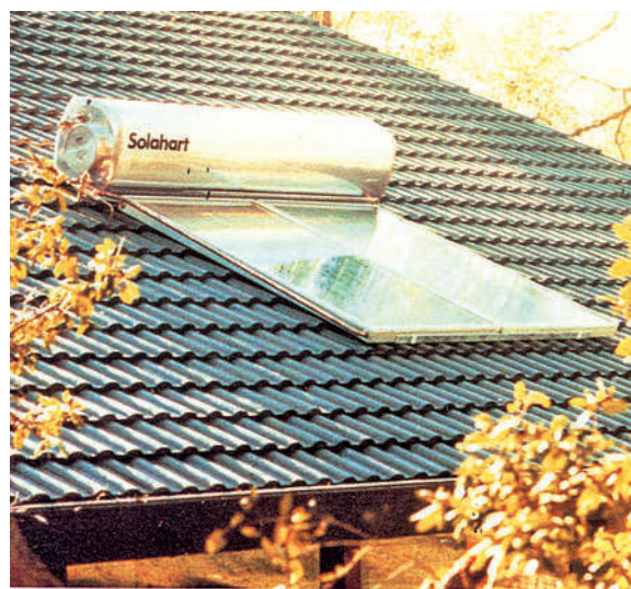
Figure 23. Solar water heater fitted on the roof of a house.
