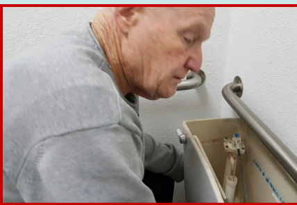
Chuck is repairing the toilet in the upstairs ladies restroom.
