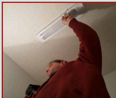
Mark repairs the light in the upstairs utility closet.
