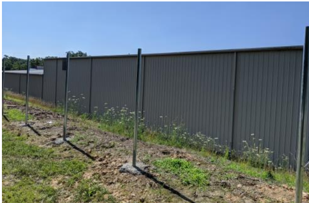
Steel posts were cemented into the ground. Photo by Penny Jost
