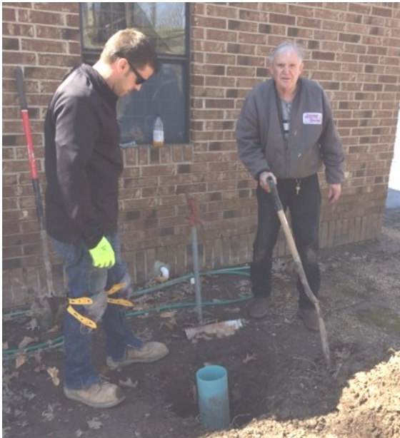
Chuck is assisting with the repairs to the water line.
