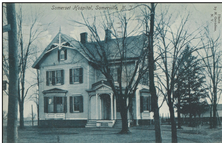
Chelsea House at 350 E Main St, Somerville, was the location of the first Somerset Hospital.
