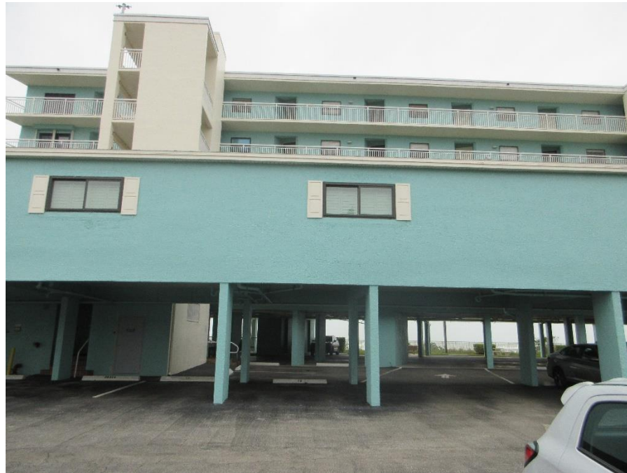
Photo #5 – East Elevation of Neighboring Building.
