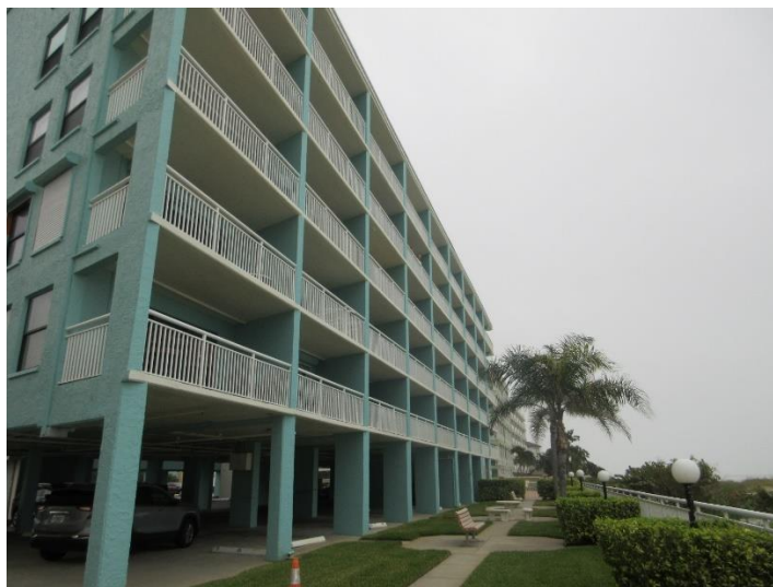
Figure 1: Northwest Overview of Building
