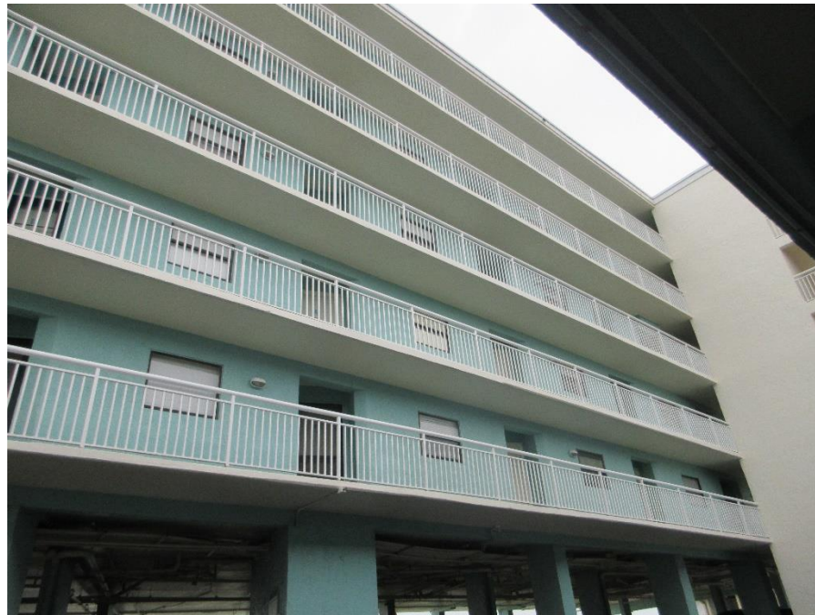
Photo #4 - East Elevation of Building.
