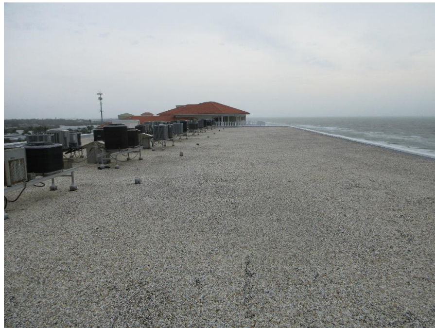
Photo #6 – Southwest Overview of Tar and Gravel Roof.
