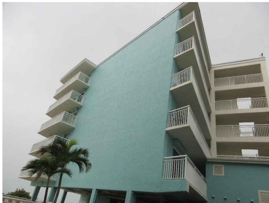
Photo #2 - Southeast Elevation of Building.
