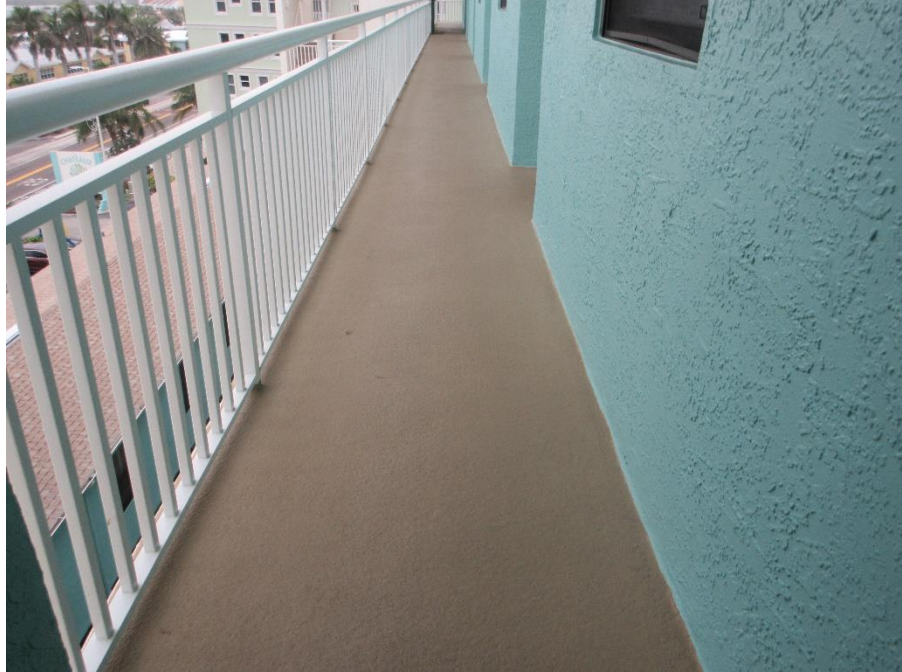
Photo #21 – Overview of Walkways Deck Coating
