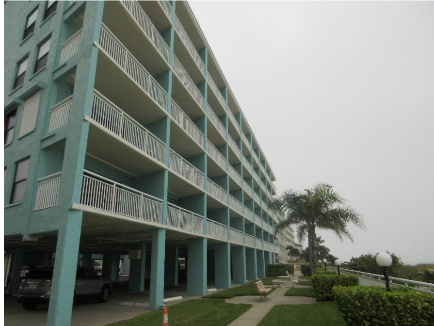
Photo #3 – Northwest Elevation of Building.
