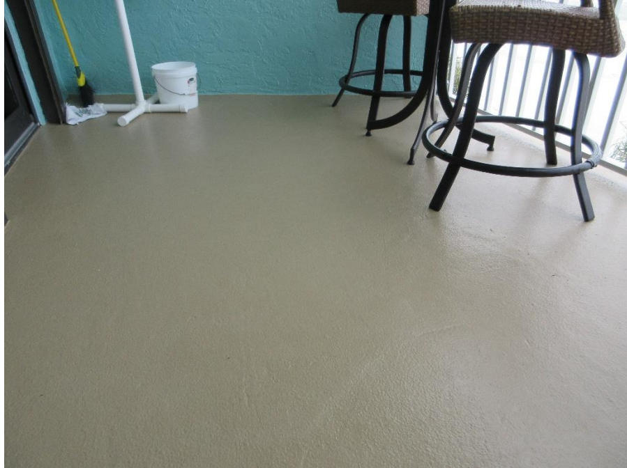
Photo #15 – Newly Painted Slab Deck at Unit #308.
