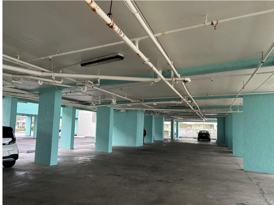
Photo #29 – Overview of Underbuilding Parking (TYP.)
