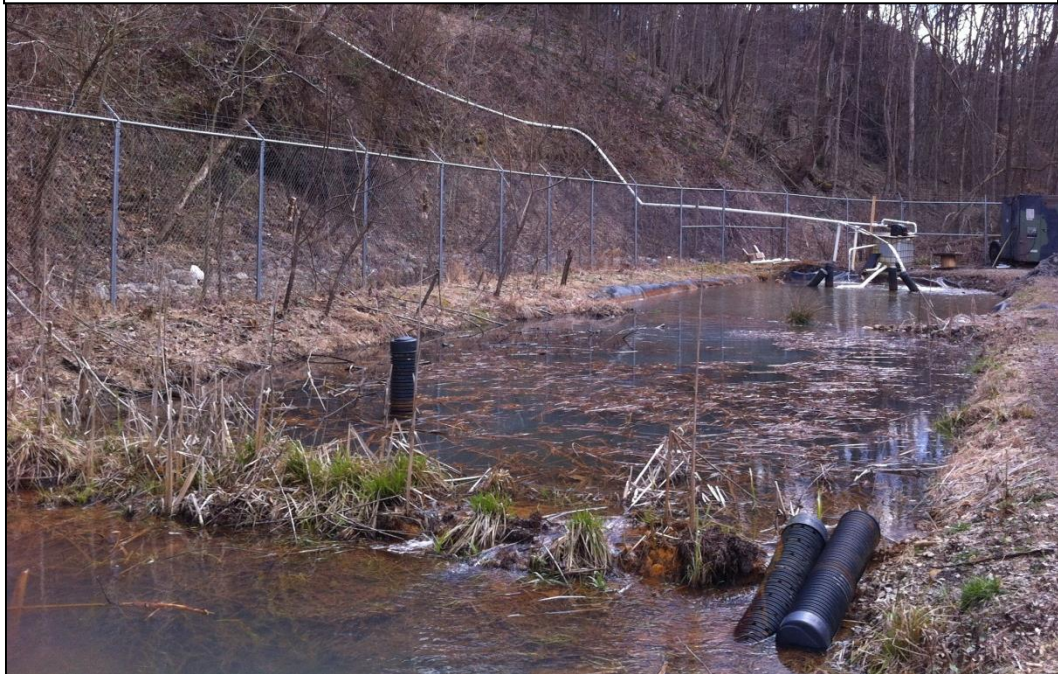
Figure 12 Present state of Lower Mainstem treatment system; hillside seep has been rerouted to head of the treatment. It is piped through generator and limestone diversion well before entering the system.
