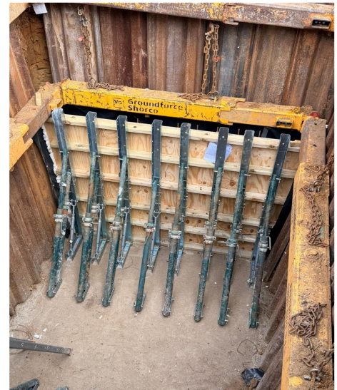
Super-Form Large Bracket, joined with large Upright for 2m pour height
