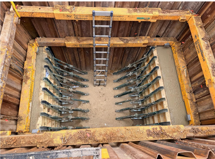
Super-Form Large Bracket, joined with large Upright for 2m pour height
