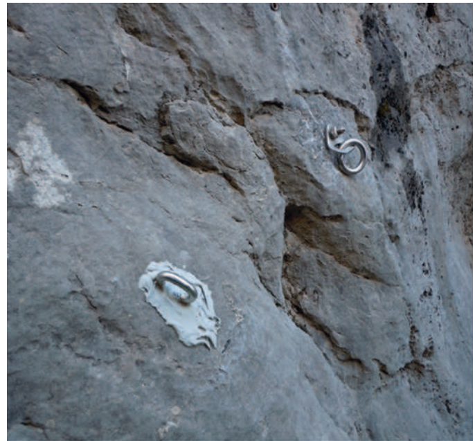
FIGURE 56-41 Standard canyon anchor expansion bolt (right) and glue-in bolt (left). (Courtesy Giacomo Strapazzon.)
