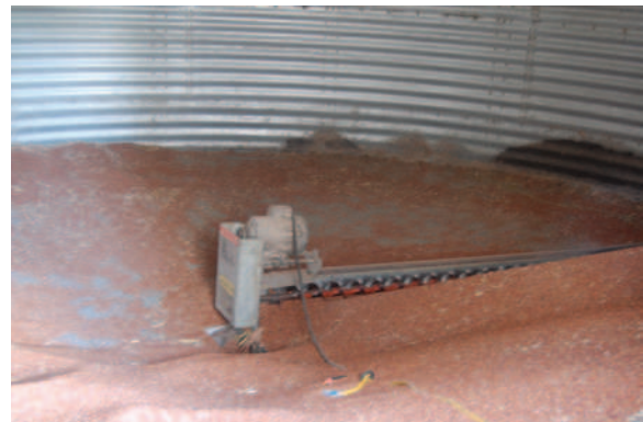
FIGURE 37-6 Auger inside a grain silo. (Courtesy of Mark Brandenburg, MD.)
