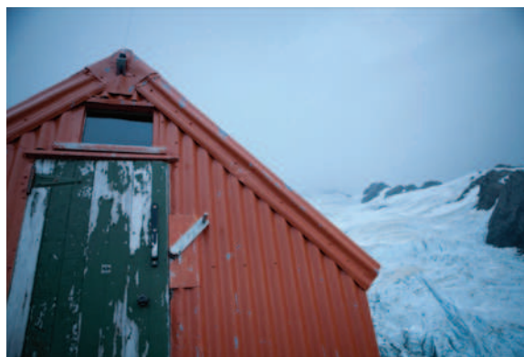
FIGURE 29-11 Constructed wilderness shelter. (Courtesy Haley Buffman.)
