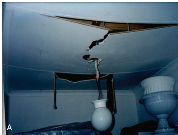
FIGURE 5-20 Damage to the ceiling (A) and internal wall (B) of the clubhouse in Figure 5-19 with resultant damage to the electrical and electronic devices connected to the electrical system. (Copyright Ian R. Jandrell.)
