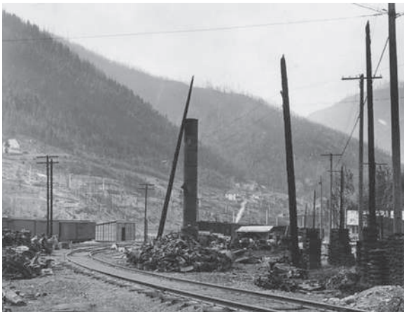
FIGURE 14-10 Burned ruins of the foundry in Wallace, Idaho, furnish mute testimony to the destructive force of the 1910 fires. The cottage on the terrace was the only one left standing in that part of town. Of the 85 people reported killed in the “Big Blowup of 1910,” 78 were firefighters. (Courtesy USDA Forest Service; photo by R.H. McKay.)
