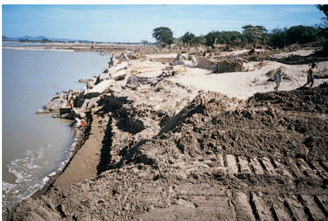
FIGURE 85-16 Aftermath of Hurricane Mitch in Honduras in 1998. (Courtesy Paul Thompson, InterWorks.)
