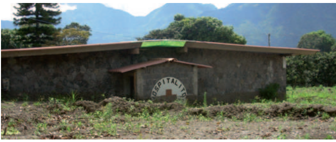
FIGURE 85-14 Former hospital in Santiago Atitlán, Guatemala, buried during mudslide. (Courtesy Paul S. Auerbach, MD.)
