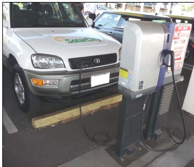
Figure 5-11: Electric Vehicle Charging Station (Photo courtesy of State Farm Vehicle Research Facility)
