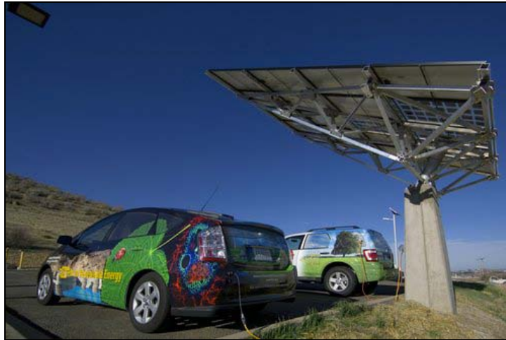
Figure 5-10: Outdoor Solar Power EV Charging Station (Photo courtesy of NREL Photographic Information Exchange)
