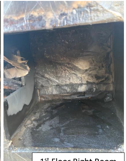
1 st Floor Right Room
