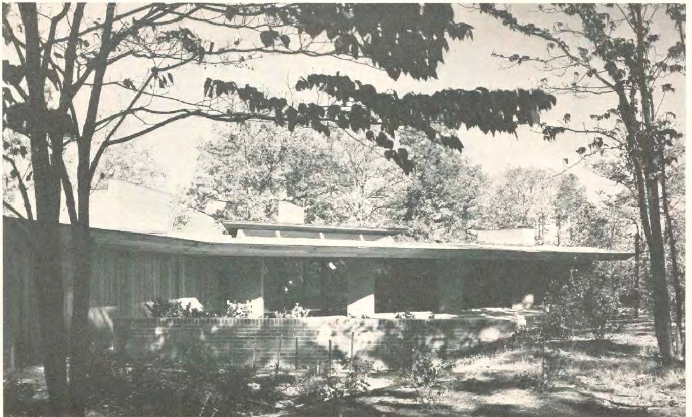
Left: general view of entrance side of house seen from drive. Service wing at right, bedroom wing at left. Below: main entrance, with skylight over dining area. In foreground, terrace outside bedroom wing, separated by brick wall from entrance court
