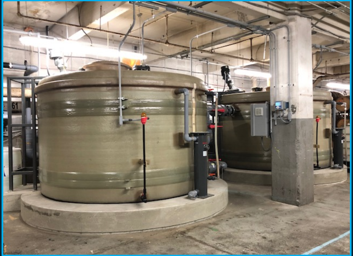
EQUALIZATION TANKS SET IN PLACE
