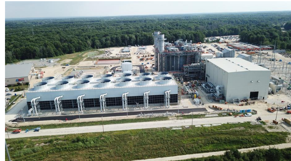
Lordstown Energy Center Ohio – 1 GW Natural Gas
