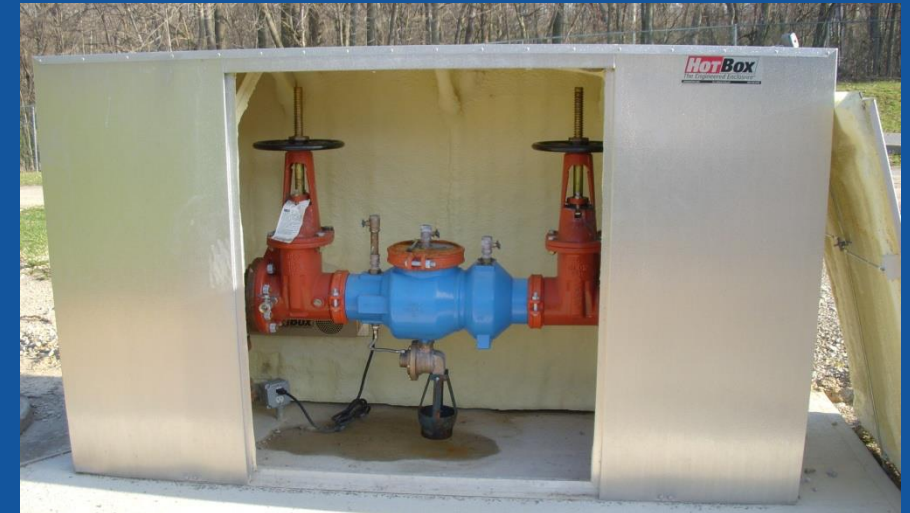
Reduced Pressure/Detector Assembly
