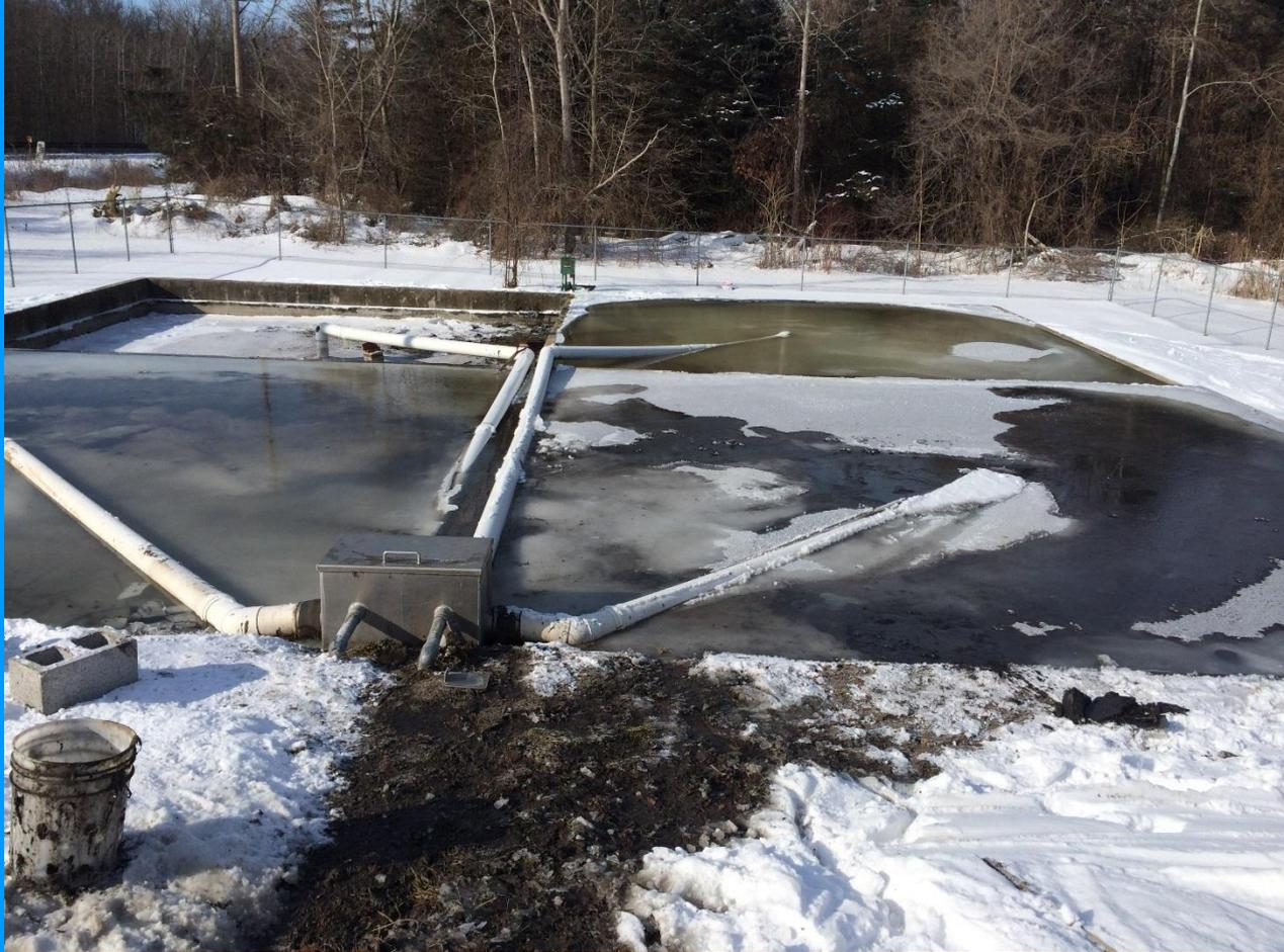
If you have EQ, pump clear water back to the EQ to speed drying times
