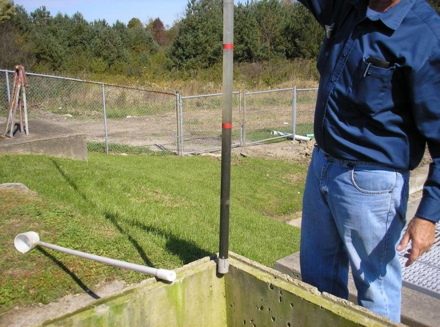
Check the sludge amounts in the dosing tank several times per year and clean it when needed, especially if the sand filters have just been covered with solids.
