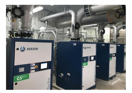
Motor Cooling Air Ducting Heat Recycle Option (Cold Weather) 902btu/min per blower (200hp)
