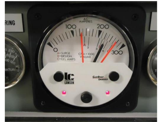
Ammeter readings above design
