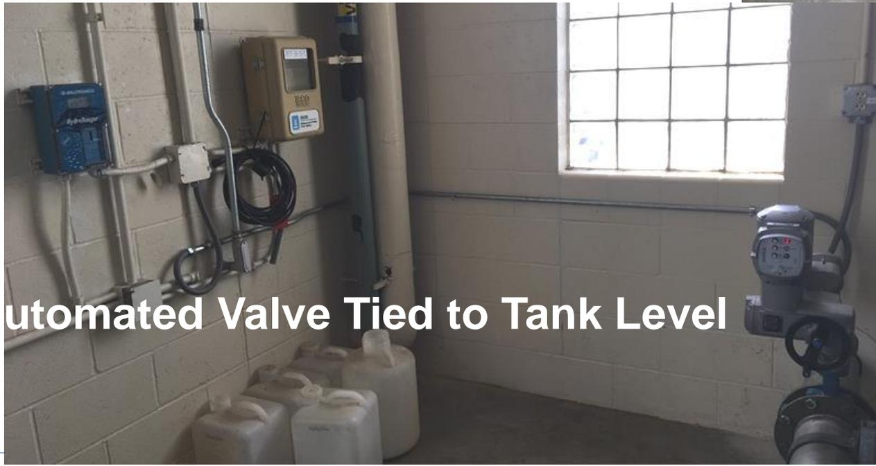
Automated Valve Tied to Tank Level
