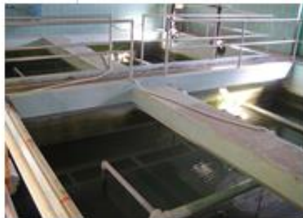
Water Plant—Gravity Filters (1966-2013)
