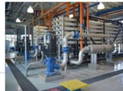
RO Membrane Softening —2013
