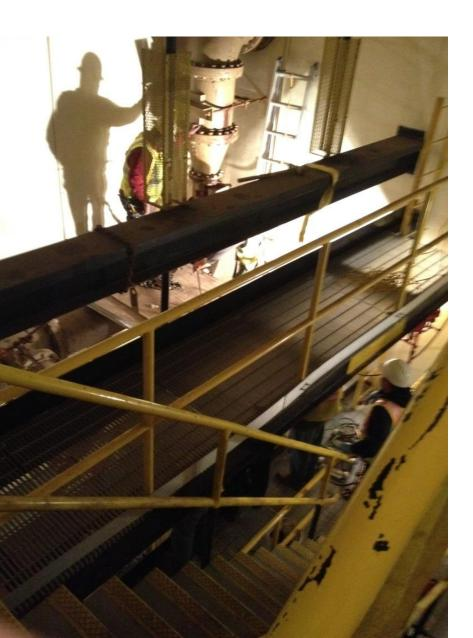
2:45 AM - Force main is finished draining and Hoffman Brothers starts repairs and Clean Earth and Terra are still pumping sewage and manually hauling it and dumping in a manhole downstream
