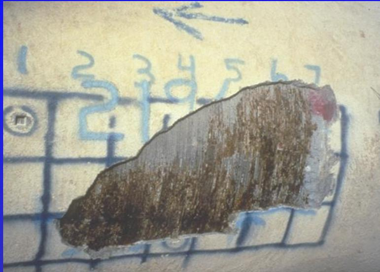
Corrosion of pre-stressed concrete cylinder pipe (P.C.C.P.).
