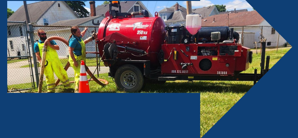
Service-Line Verification Pot-Holing Demonstration RCAP Field Day, 06-11-2024
