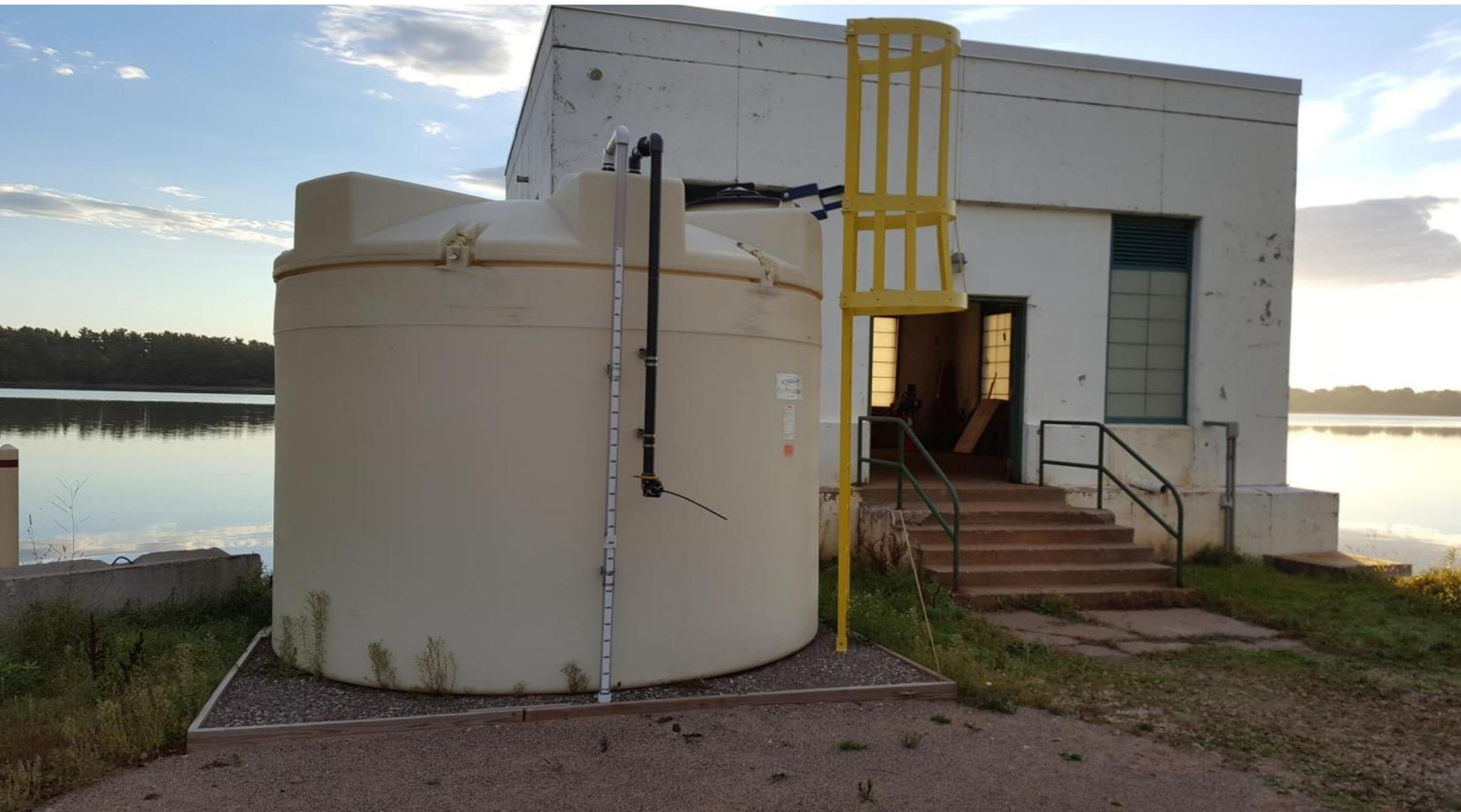
**Bulk storage tank for EarthTec QZ -- 5,500 gallons**
