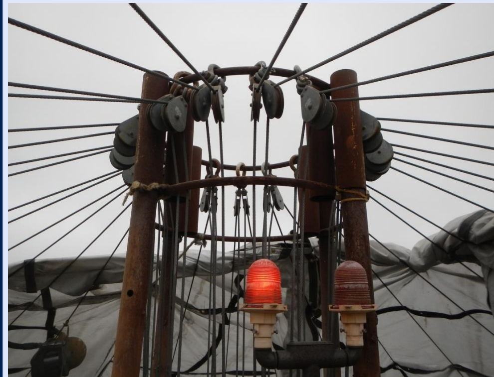
Center Pulley Assembly
