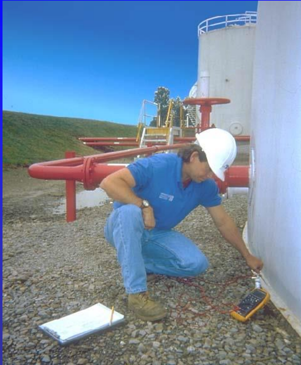
Annual Cathodic Protection Survey
