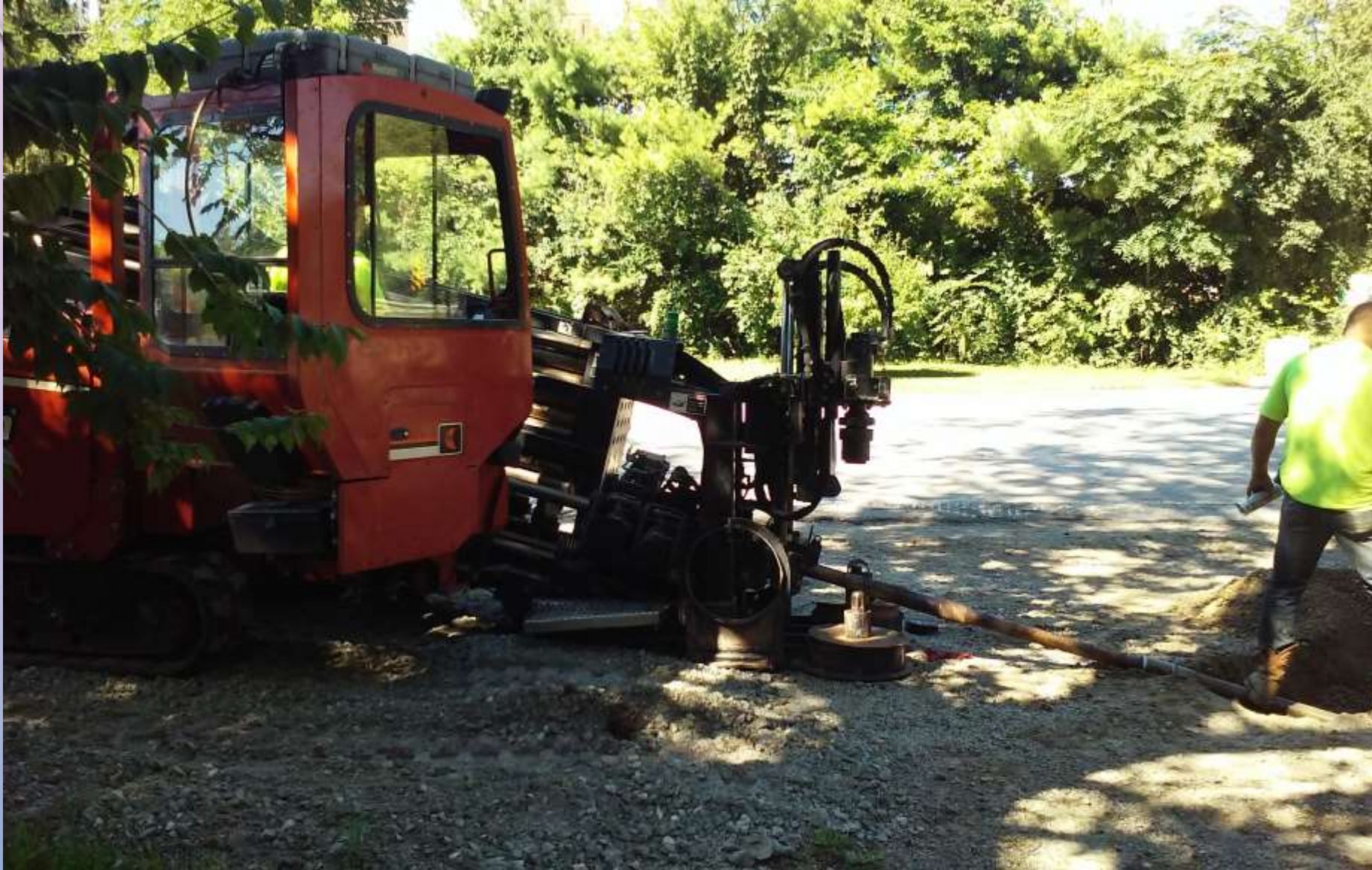
Setting up bore for Mud Run
