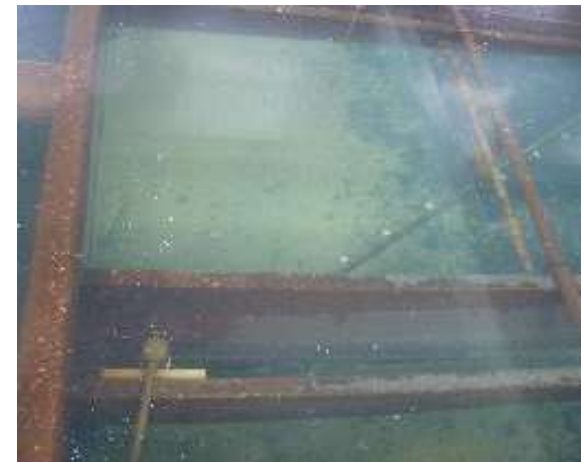
Clarification and sedimentation are important to successful filtration
