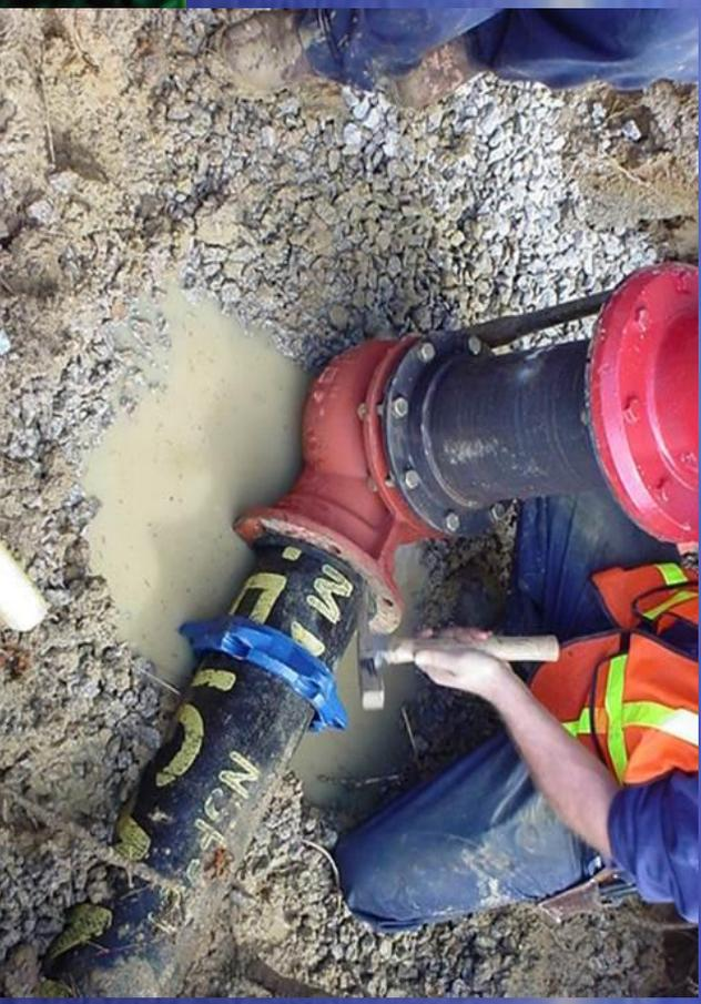
\* Note the lack of proper thrust blocking around the shoe.
