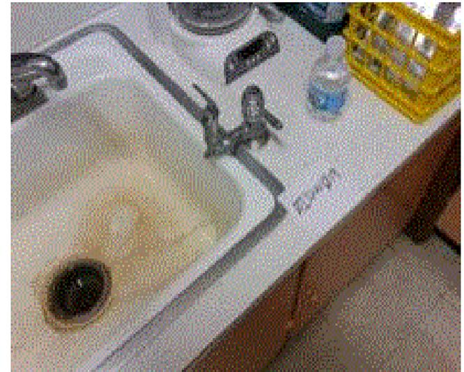
Replacement of this bubbler tap and its connecting plumbing with lead-free materials will significantly reduce lead exposure at this location. If replacement is not currently feasible, sample results indicate that flushing this tap for three minutes following periods of stagnation is likely to reduce lead concentrations and lead exposure.
