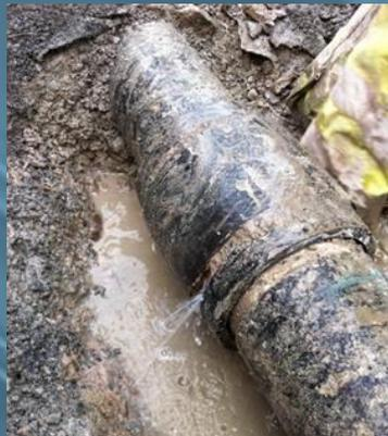
Ductile Iron Push-On Joint
