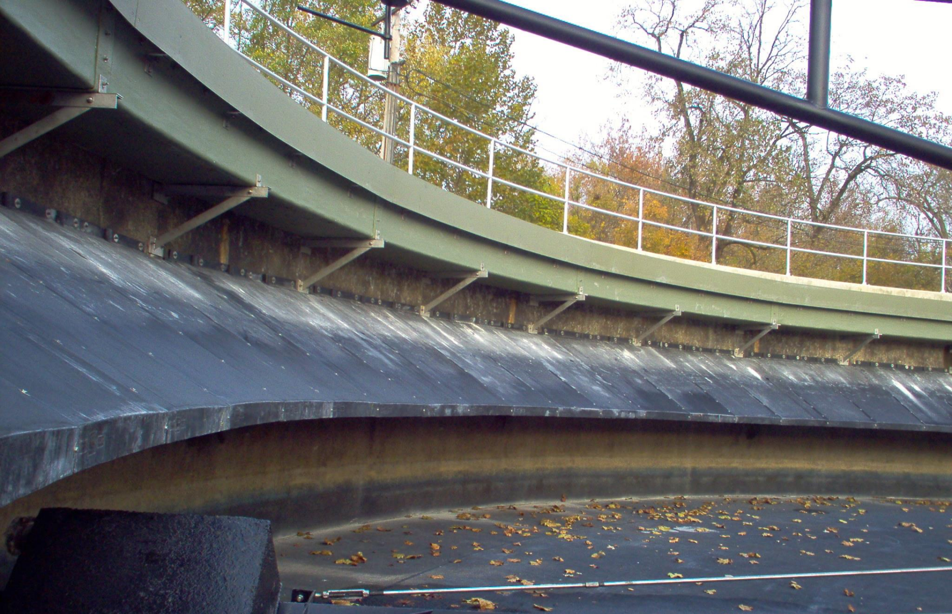
30° LARGE PROJECTION BAFFLES AT AKRON, OH
