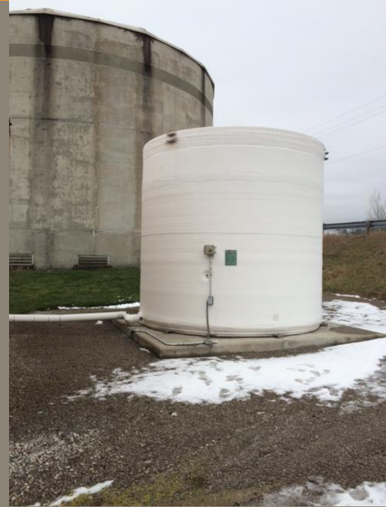
Alum Tank at the Napoleon WWTP
