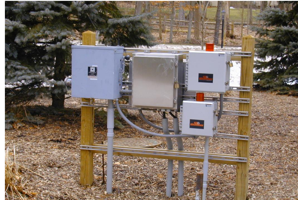
Dry Well Lift Station
