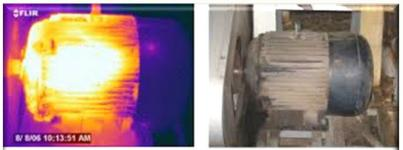
Above thermal and daylight images show a three phase motor which has overheated. Power quality analysis proved condition was caused by negative sequence harmonics.
