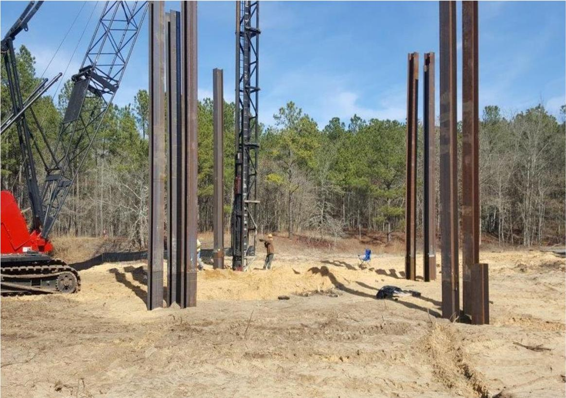
Piles (steel or auger cast piles)
