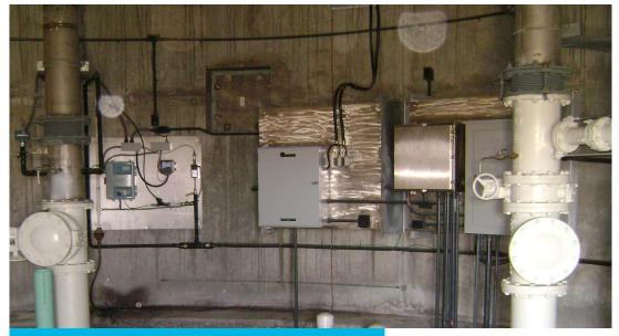
Separate Inlet/Outlet Pipes
