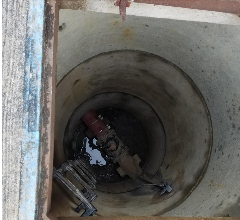
Figure 1: Located in pit
