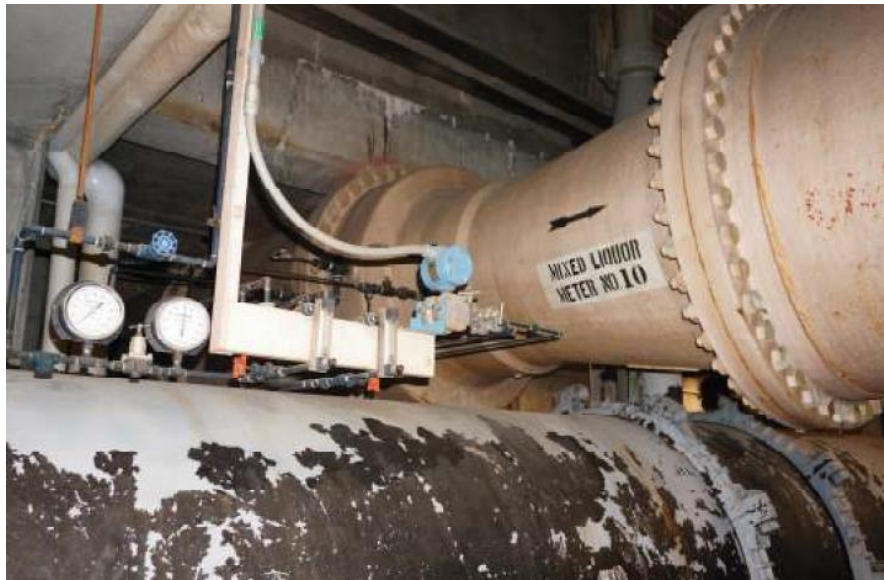
Figure 1: Existing 48" Venturi meter
