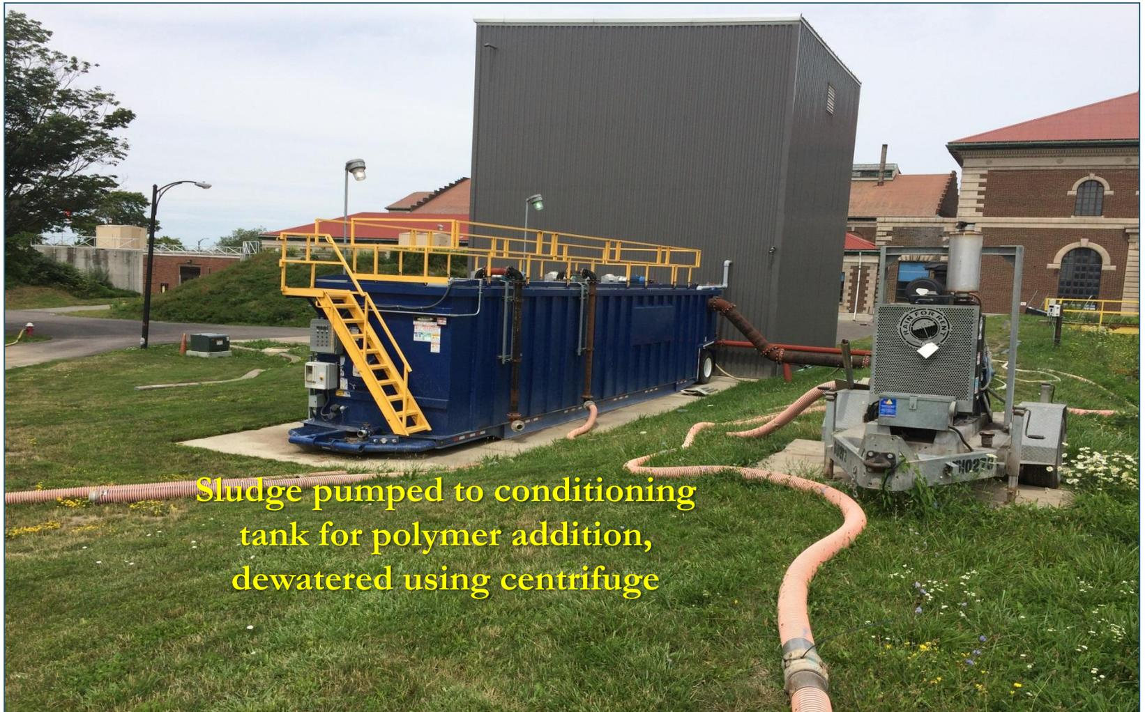
Sludge pumped to conditioning tank for polymer addition, dewatered using centrifuge
