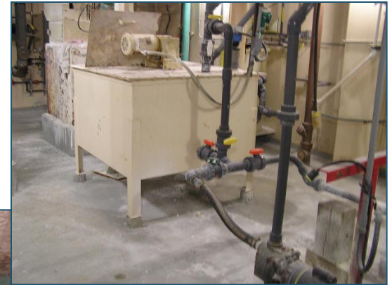
Alum, carbon fluoride, lime fed to raw water channel upstream of rapid mix
