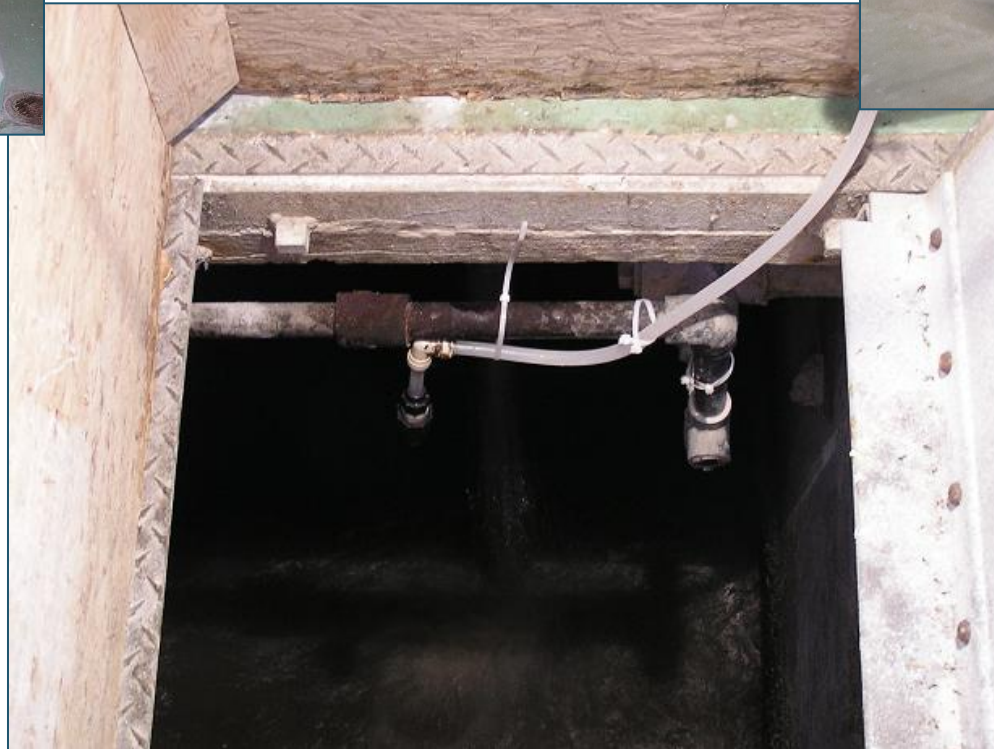
Alum, carbon fluoride, lime fed to raw water channel upstream of rapid mix
