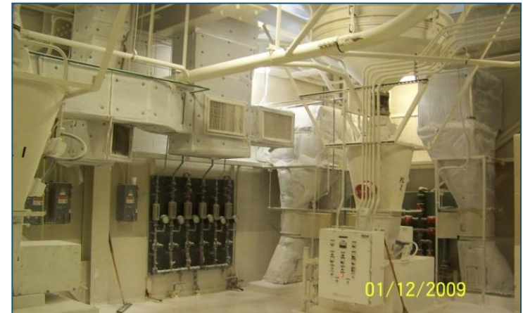
Dewatering lime feed
