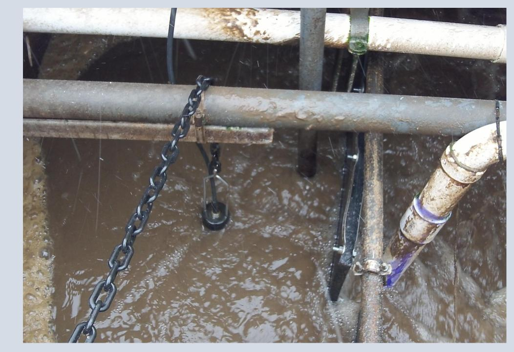
Aeration Tank Baffle Installed to **Prevent Short** Circuiting from Splitter Box to Clarifier
