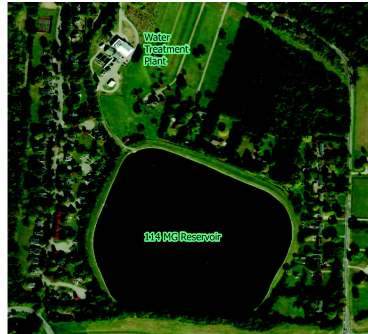
City of Franklin's WTP and Reservoir
