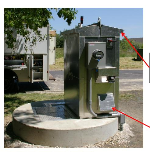
Air intake under the roof overhang 60" above grade
